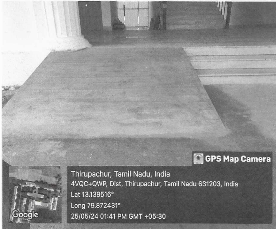
Ramp facility from A-black front side at SVCET
